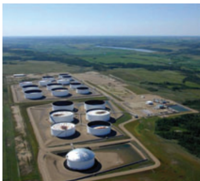
The new tanks, with coatings and linings performing well Courtesy of Enbridge
