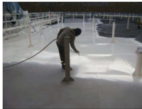
Worker spray painting roof Courtesy of Park Derochie Coatings Ltd.
